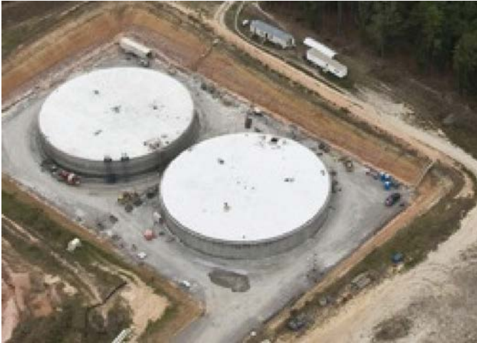
Figure 1.2 Low-activity waste disposal in grout at the Savannah River Site shows volume of waste that may require long-term stabilization. Courtesy of Dan Kaplan
